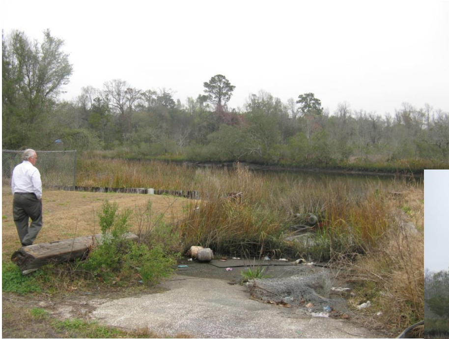
Derelict Boat Ramp
